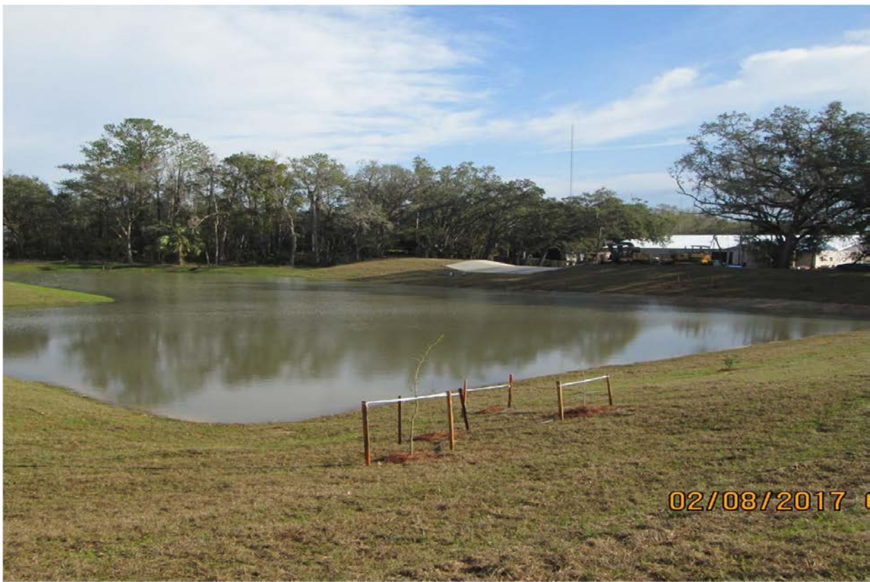
GOOD NEIGHBOR TRAILHEAD AREA REGIONAL STORMWATER PROJECT (2/08/2017)
